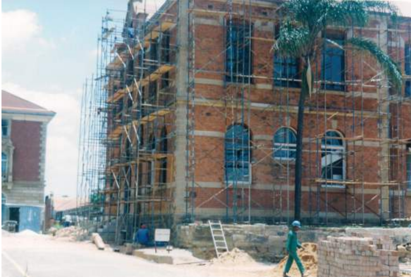
Figure 9-6: The restoration of the Machine Building by AJ Construction
