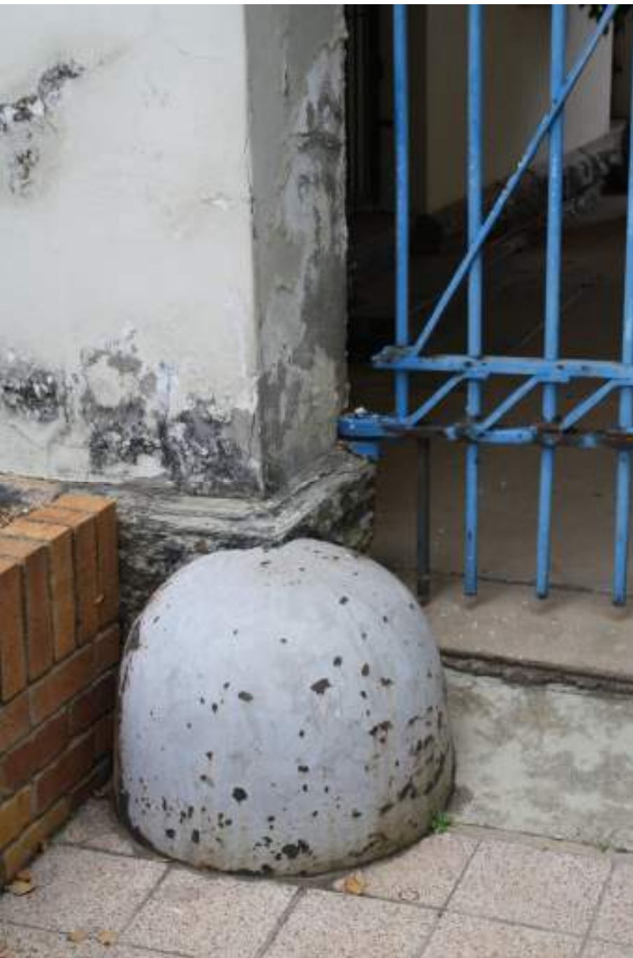
Figure 5-2: Cast-iron balls used to prevent damage to the cannon and wagon stores still in place at the entrance to the northern cannon and wagon stores
