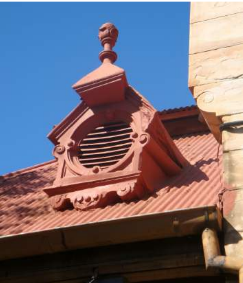
Figure 6-7: The glamorous roof shutters fitted to the officers' residences
