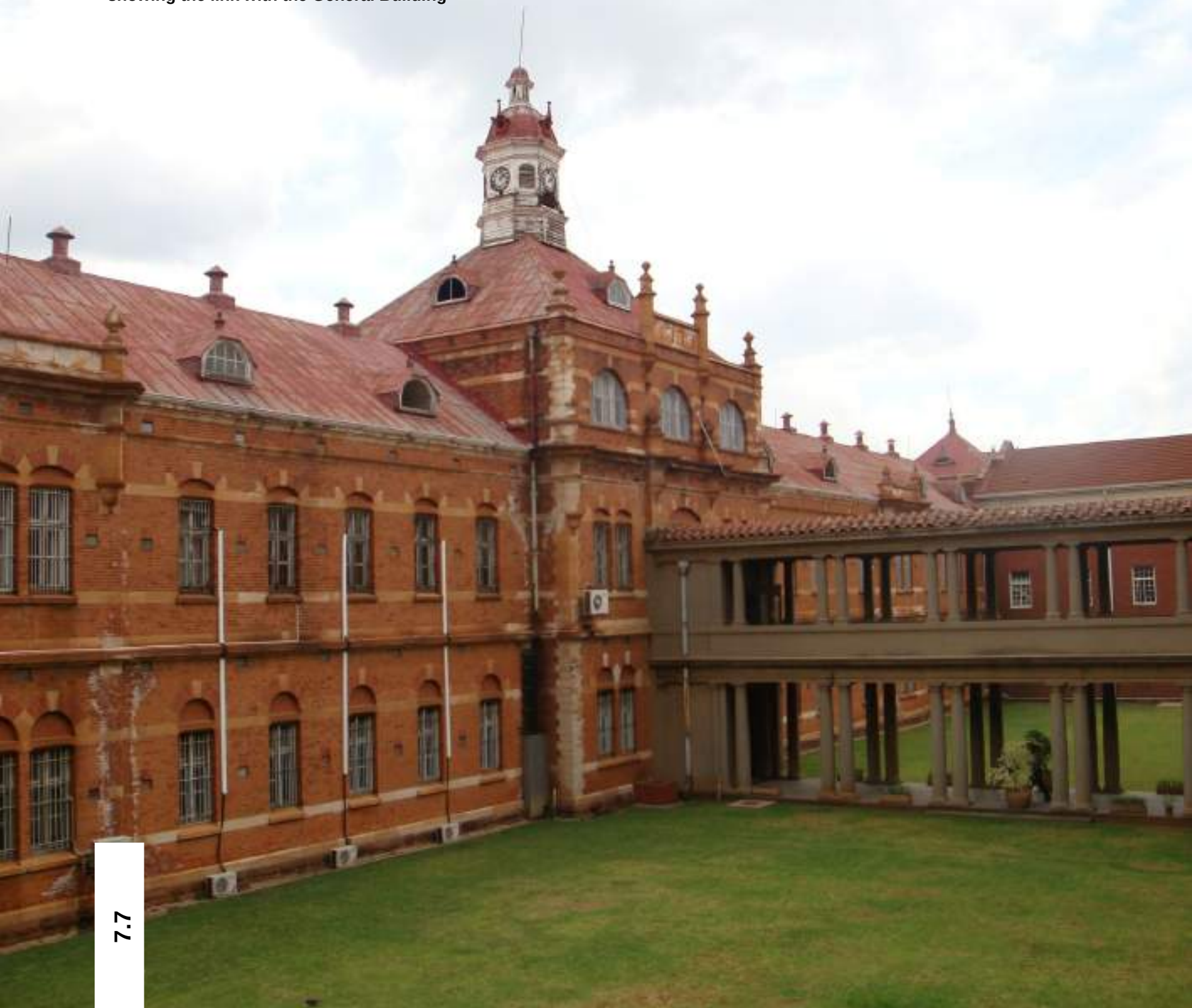
Figure 7-7: Modern-day entrance to the barracks showing the link with the General Building
