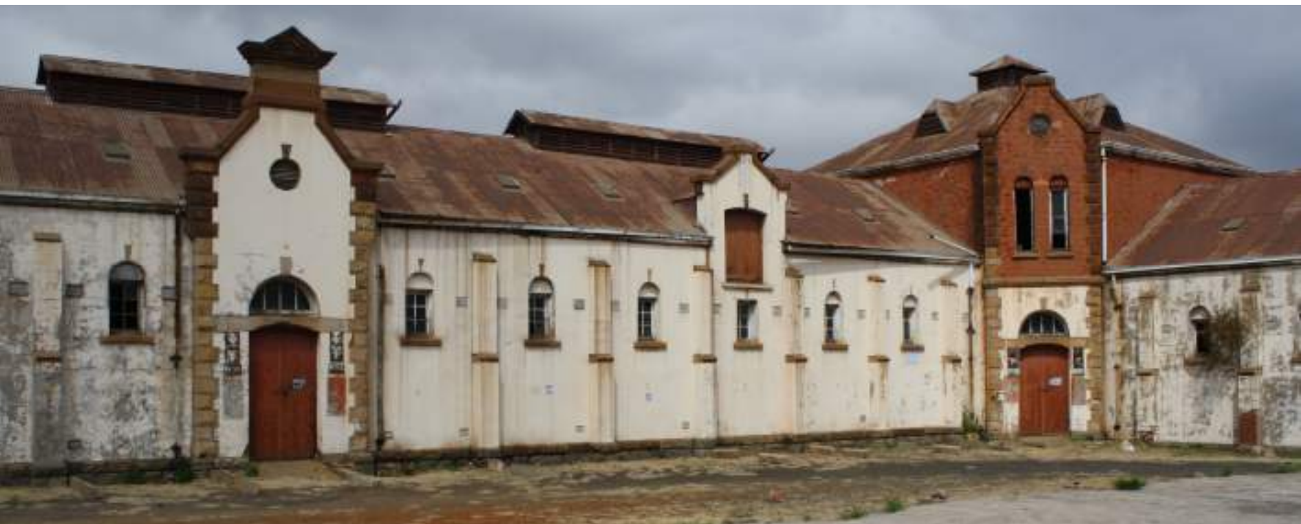
Figure 3-13: The only original roof shutters remaining after the 1948 hail damage resulted in all the others being replaced
